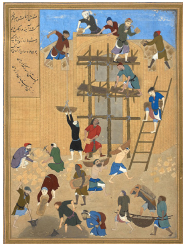
Construction of the fort of Kharnaq Kamal ud-din Behzad
